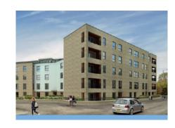
Sigmat were appointed by award winning Scottish developers MNM to manufacture, assemble and install the steel frame superstructure, solid concrete floors and allow for a basement car park. Large glazed windows were part of the design to allow natural light to enter the open plan apartments.
