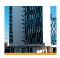
The building contains 361 bed spaces in 36 clusters, including 217 studio flats. With 11 floors of light gauge frame sitting upon a first floor podium, Sigmat believes this is currently the UK's tallest completed light gauge steel frame building. The Sigmat team completed the multi-level scheme in just 17 weeks.
