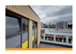
Sigmat designed and installed an 8-storey light gauge frame for the student accommodation block at the heart of the scheme. The installation took just 20 weeks.
